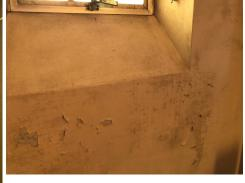
The dual issue: mould and peeling \( \backsquare \) paint
